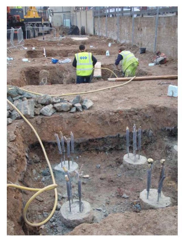
Plate 3. Phase 2. Ground reduction around pile caps (through made-up ground)
